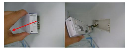
Unplug the connecting wire and replace the control box
