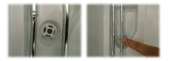
**2/4** Wrap the valve with aluminium adhesive tape on the back of the appliance. Then re-assemble the WOT condenser to the back of the appliance ensuring the integrity of the brazing
