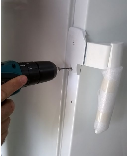
4. Drill a new hole in for the lower fastening.
