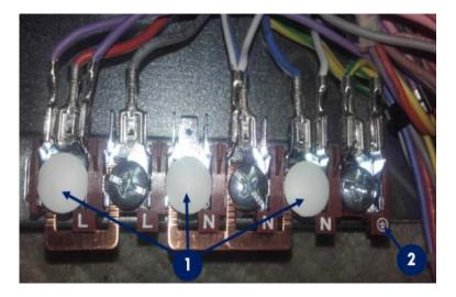
Future Production will eliminate these Blanking Buttons. When removal is required for service operation note the correct connections. The connection plate is adhered to the rear panel.
