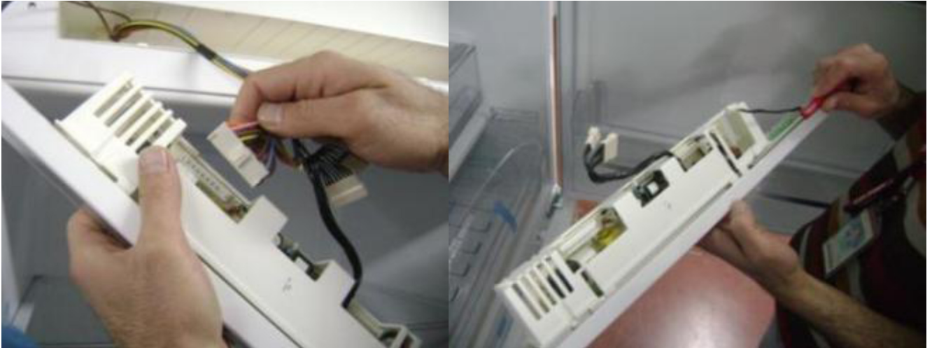
7. Connect the mainboard connector and then place the mainboard group on housing.
