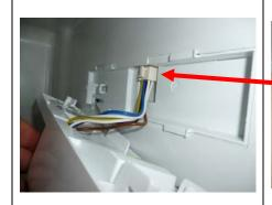
4.Remove the capillary from plastic tube
