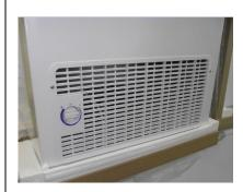
2.Remove the screws of the side cover then remove the cover gently
