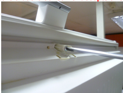
1. Screw out the lock
