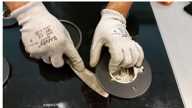
2. Remove the old cover using a tool with rounded edge not to scratch the glass surface
