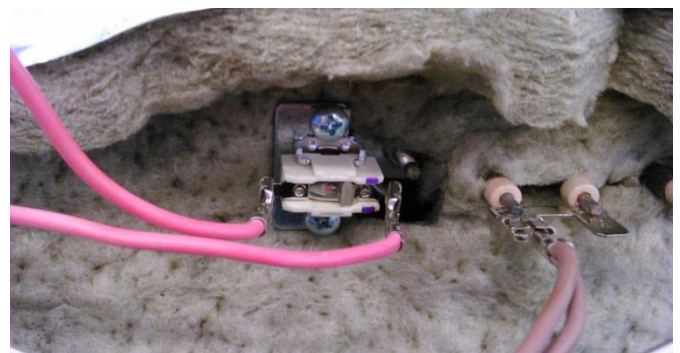
2. New thermostat after exchange
