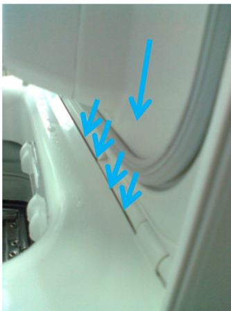
Water dripping way.
