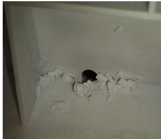
6. Clear the holes and appliance from drilling leftovers.
