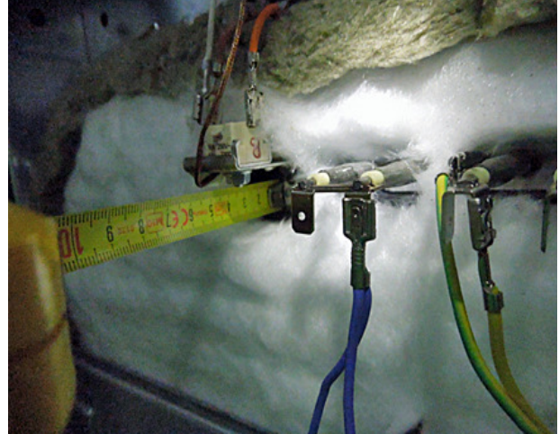
2.3. Example of incorrect insulation fitting – large distance between the insulation and cavity may influence thermostat operation
