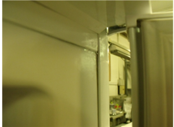
6. Make sure the corners are filled properly.
