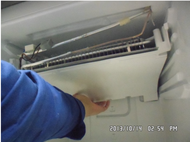
7. Pull the evaporator battery away from back wall.
