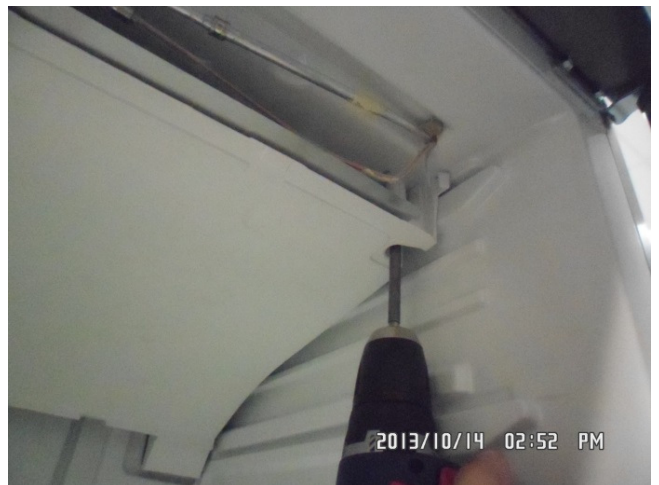
30. Screw evaporator battery to compartment ceiling.
