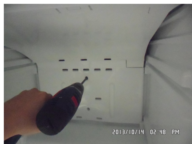
2. Unscrew air duct cover.
