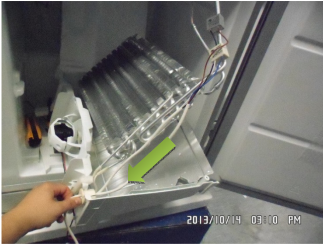
21. Adjust the wires (pull out few mm if needed).
