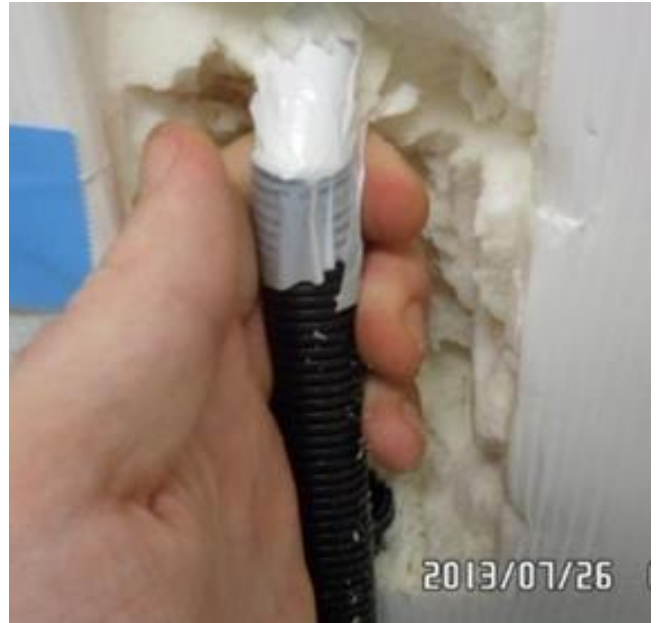
8. Fasten drain hose with adhesive tape (~10cm strip).
