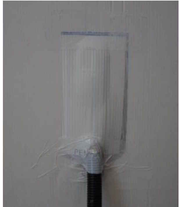
12. Bend back corrugated material and secure it with adhesive tape.
