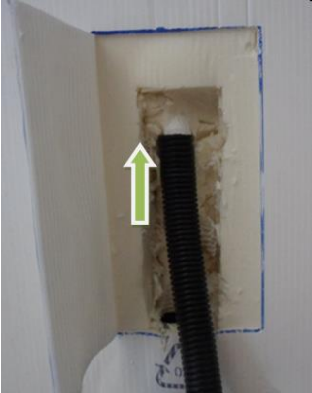
7. Attach new hose to drain channel spigot.
