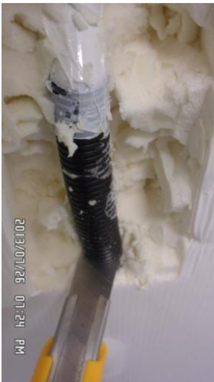
5. Remove tape securing drain hose and cut the end of hose as indicated in picture.
