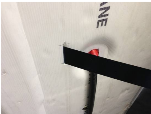
5. Insert the metal sheet without heating element in the foam
