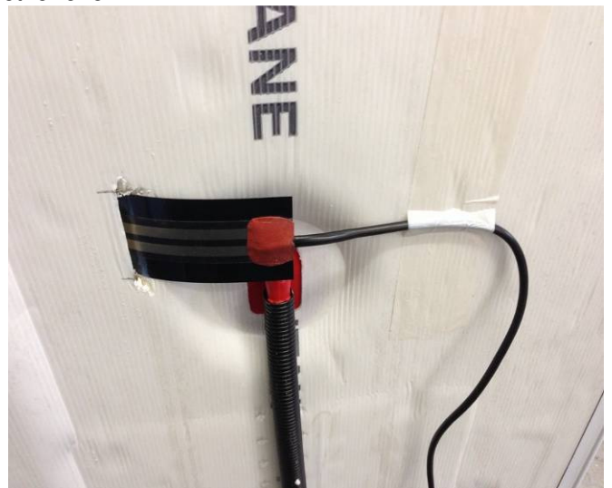
10. After positioning the heating element, remove the metal sheet and fix the cable to the corrugated material with adhesive tape
