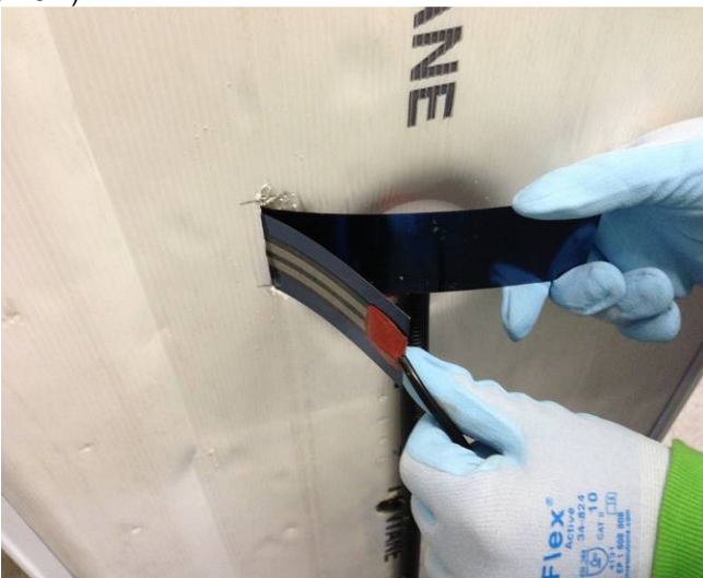
9. Take out the metal sheet without heating element
