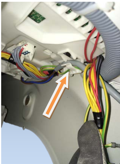
Remove the power cable from the hooks that hold it close to the board
