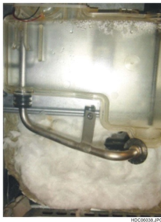
Fig. 13 : Overfilling pipe fixing detail.
