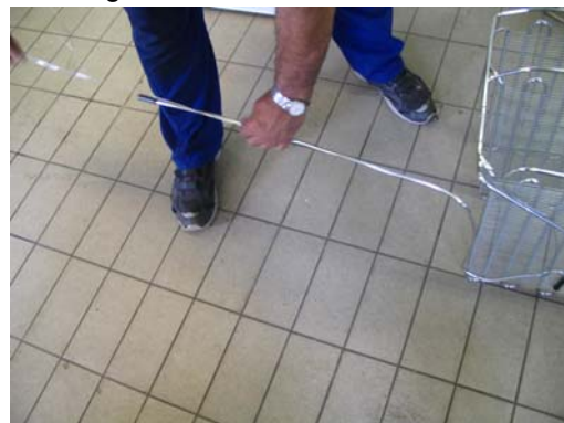
11, Straighten the suction tube of the new evaporator
