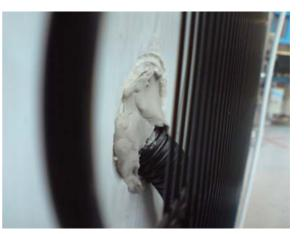
N.B. It is necessary to move the condenser sideways in order to seal the duct.
