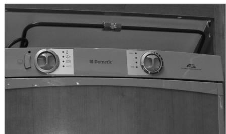
Cut-off the electrical voltage supply for 12V and 230V on the wrap connections.
