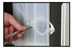
To dismount the water softener, these attachment screws are removed.
