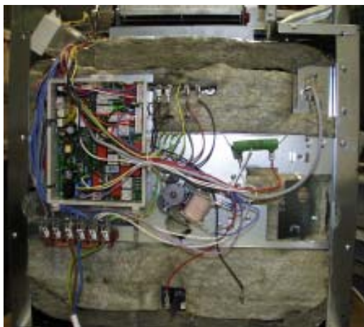
Fig.: assembly situation
