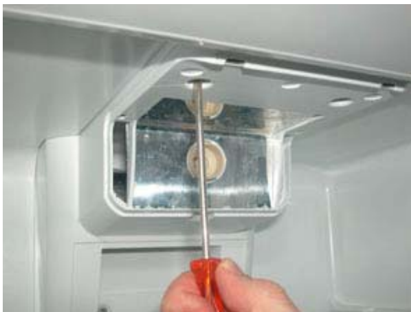
c) Unscrew the 2 upper fixing screws
